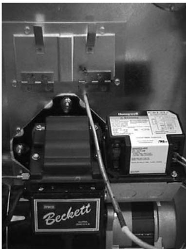
Check the oil pump pressure. Refer to Table A1, page 17, for pump pressure settings.
