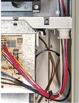
**4. New Wiring Harness** - was revised to make removal and service of the blower assembly quick and easy. The plugs are matched to ensure that the correct wires are replaced to the proper location when the blower is reinstalled or service is complete.
