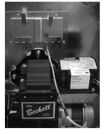
Check the oil pump pressure. Refer to Table A1, page 17, for pump pressure settings.
