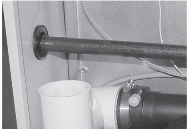
The gas piping may enter the furnace from either side. Once the routing of the gas pipe is determined, select and remove the applicable knockout and install the grommet within the hole.
