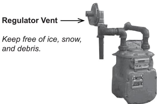
It is important for these vents to remain clear. Do not allow moisture, which could freeze, to build up in the vent. If you see moisture building up in the regulator vent, contact your gas supplier.
