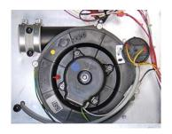
4. <u>Draft Inducer</u> –The inducer has a totally enclosed motor, which increases protection of the windings. The inducer also facilitates the mounting of the pressure switch to the inducer, which makes changing the position of the furnace easier.
