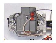
3. <u>24-Volt Gas Valve</u> – replaces the Honeywell Smart Valve II. The 24-volt valve is a universal industry standard making the furnace more service friendly and familiar to installers.
