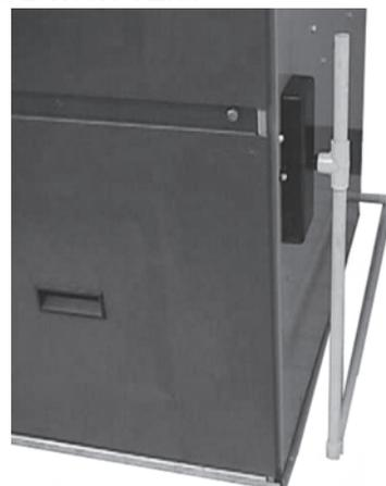
**FIGURE 27 - CONDENSATE BYPASS**
