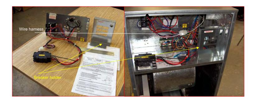
3. Install the breakers, connect power to the breakers and install the front door.
